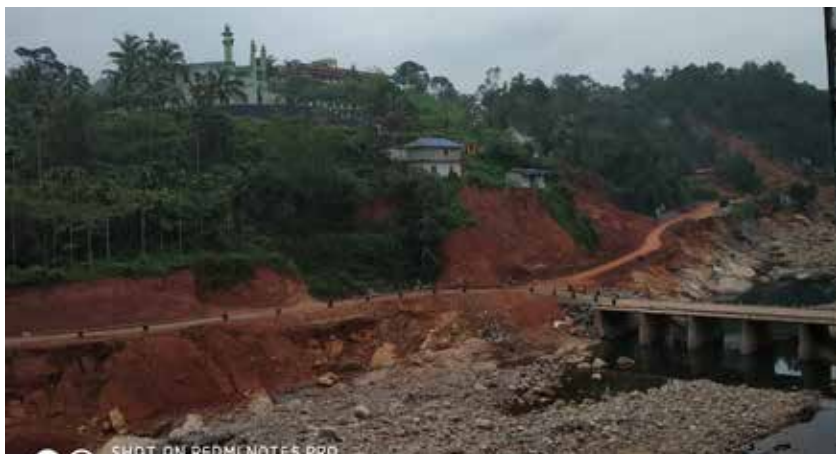
Falling rooftop : Idukki, the rooftop district of Kerala was ravaged in the 2018 floods by hundreds of major and minor landslides. The district is ecologically fragile with high disaster vulnerability.
