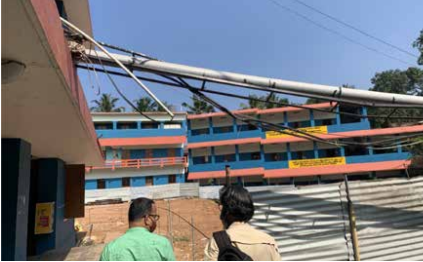
Figure 9: Rain-water harvesting pipes (Kulathummal School, Kattakada)
