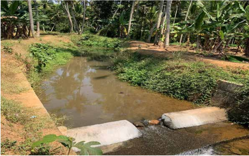
Figure 17: Check Dam to improve groundwater recharge
