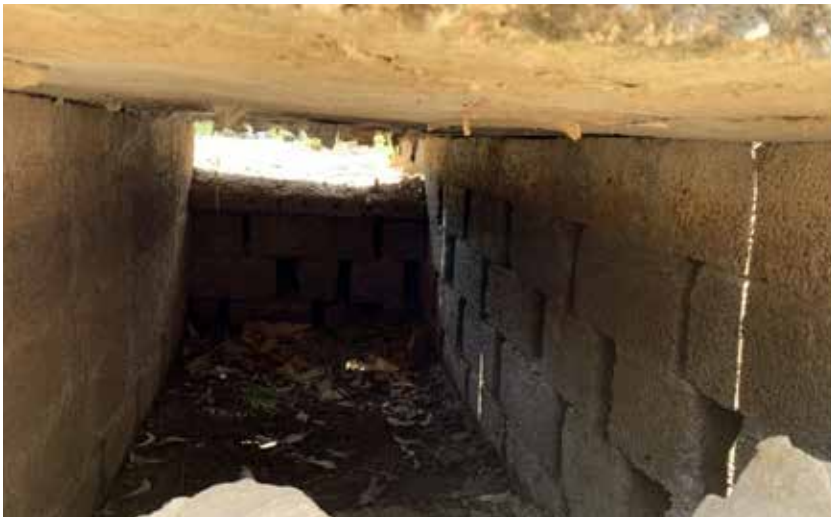
Figure 12: Roadside Honeycomb Rainwater Harvesting Structure
