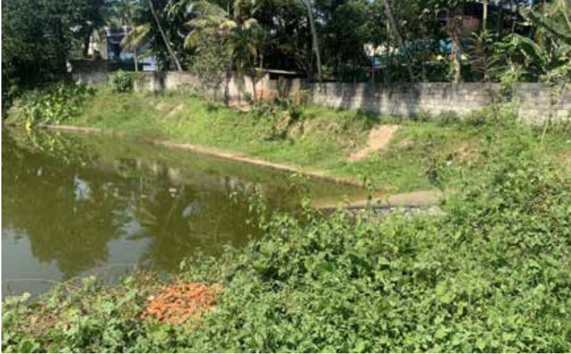
Figure 6: Side Walls of Mathrakonam pond
