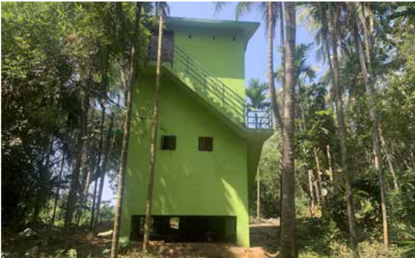
Picture 3: Pumping Station
