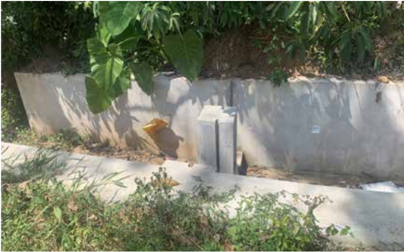
Picture 4: Regulator in Lift Irrigation Scheme in Amachal Yelah, Kattakada Panchayat
